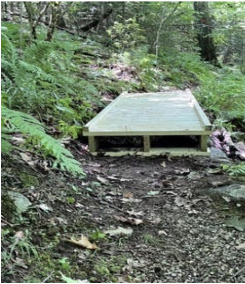
New bridge at Little River. Photo by Vanessa Noyes
